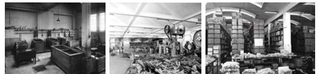
1950 Galvanising department 1955 Shearing department 1960 Shipping warehouse
