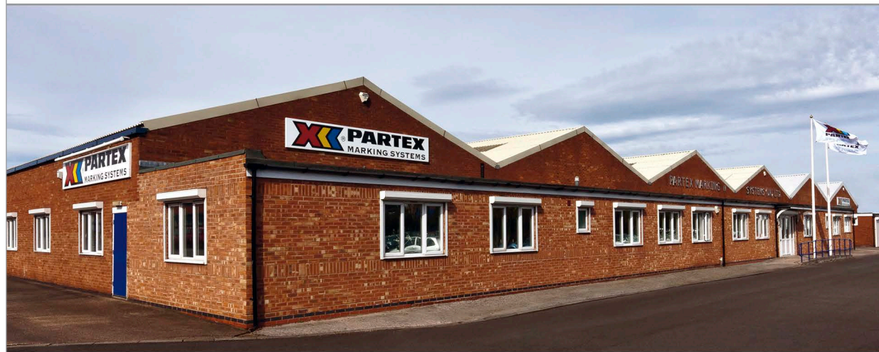
ParTex UK headquarters
